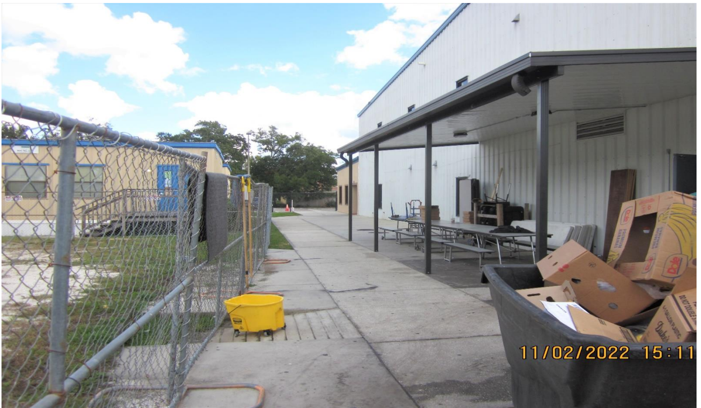
Rear main building, facing east towards the existing covered patio, the proposed patio will be behind
