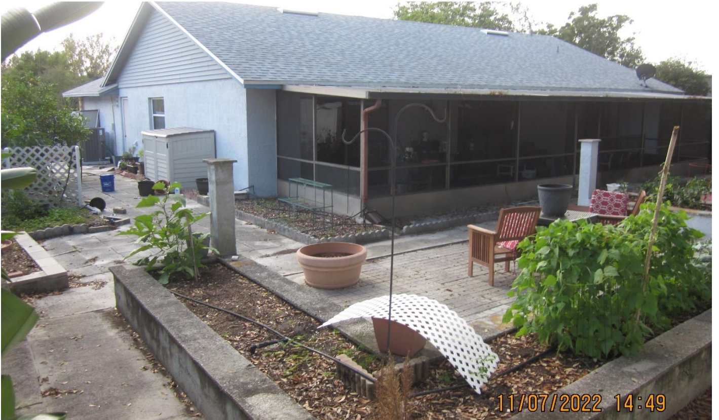
Existing screenroom facing south
