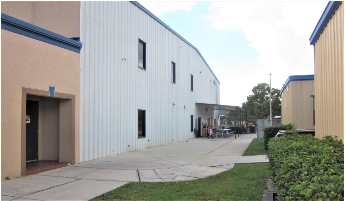
Rear main building, facing west towards the proposed new covered patio and the existing patio
