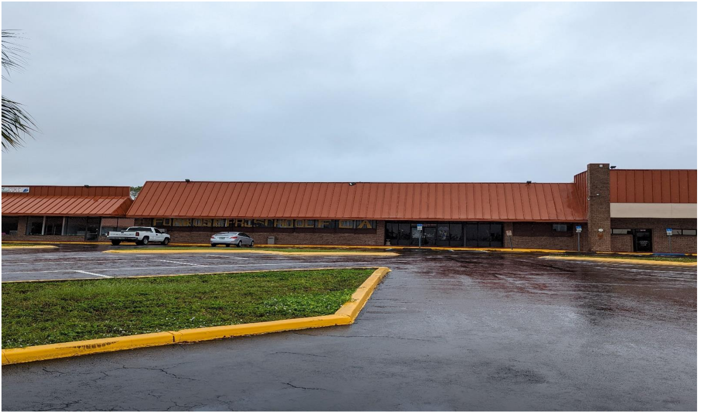
Facing south towards front of subject property
