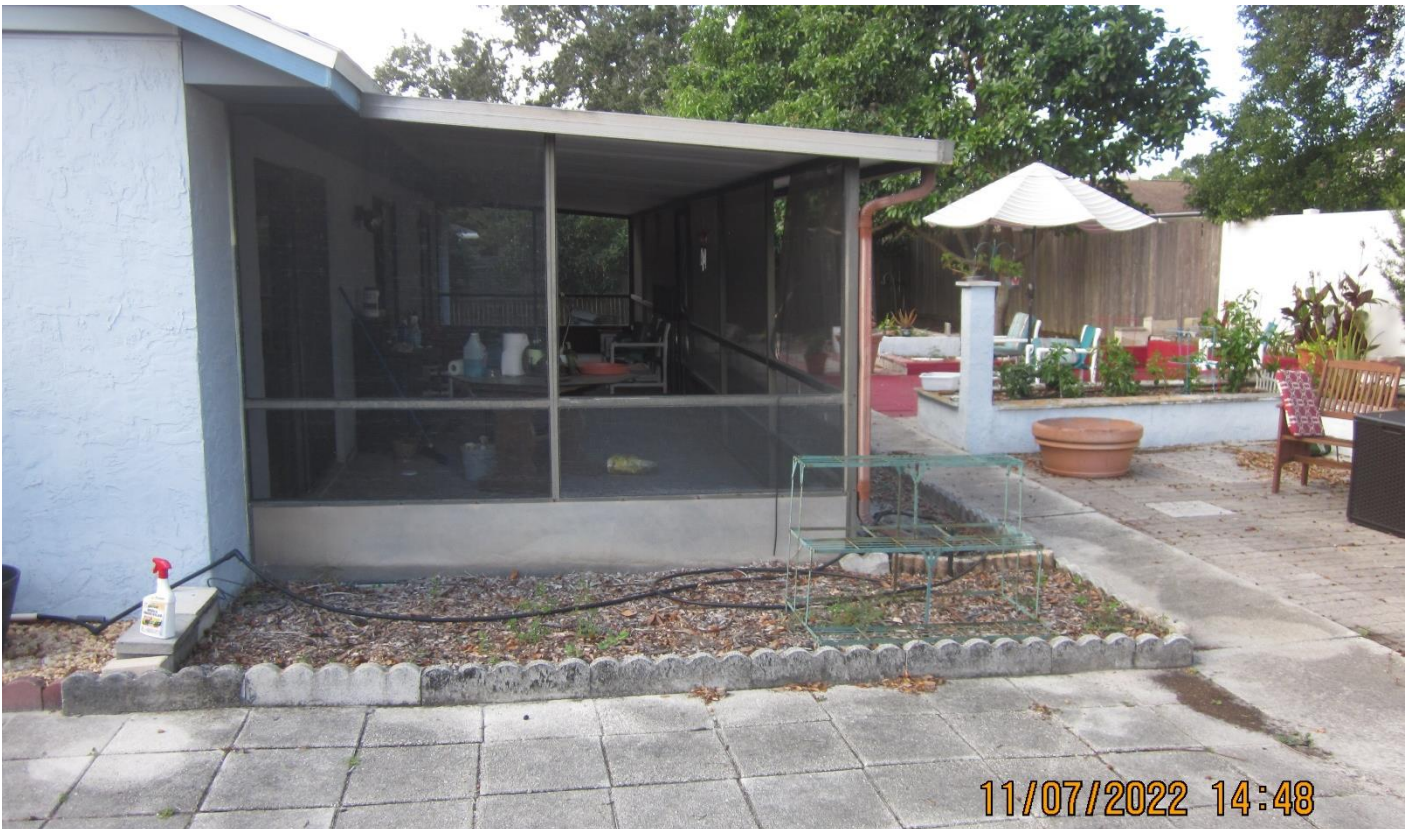
Existing screenroom facing west
