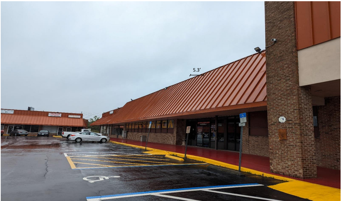
Facing east towards front of subject property
