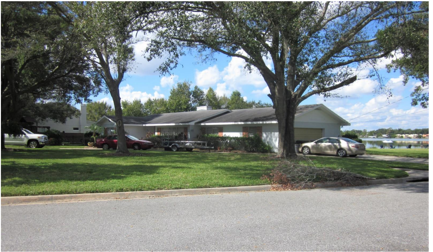
Facing northwest from corner of Ridgcrest Rd. and Troy Dr. towards front of subject property
