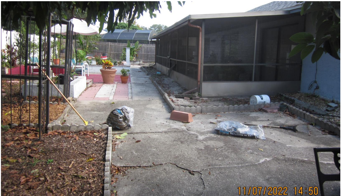
Existing screenroom in rear yard facing east
